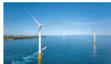
Nyuzen Offshore Wind Farm
