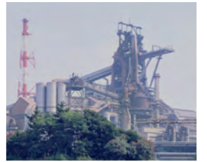
Chiba No. 6 blast furnace
