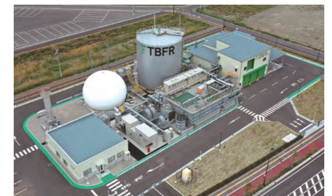
External view of plant at Tohoku Bio Food Recycle Co., Ltd.
