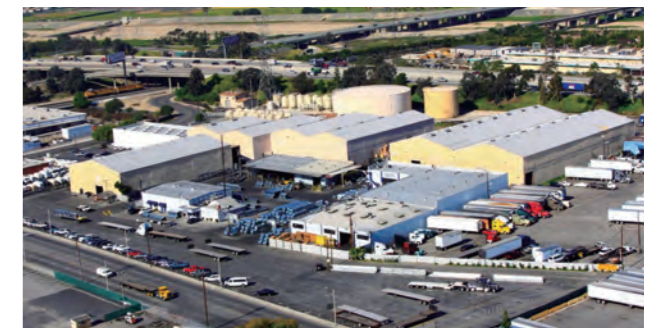
Main plant at CEMCO
