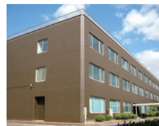
Customer Center Fukuyama
