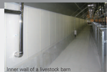
Inner wall of a livestock barn
