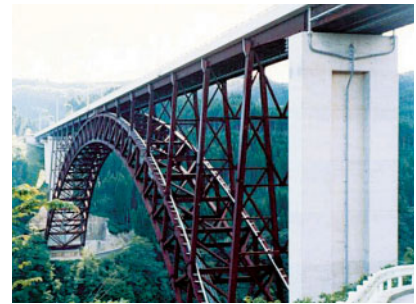
Bridge constructed using weathering steel
