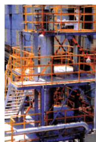
CFB test device (biomass treatment capacity: 150 kg/hr)
