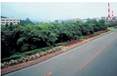
Greenbelt at Fukuyama, West Japan Works
