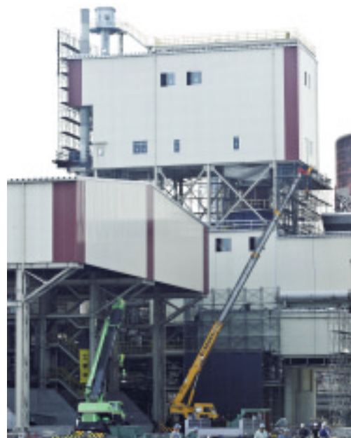
We are currently constructing a shaft furnace (height from ground= 50 meters)
