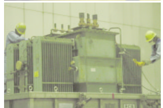
Transporting transformers at the JESCO Kitakyushu Facility
