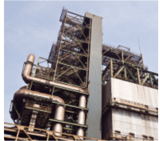
Processing equipment for gas emissions from sintering furnace: an example of the activated coke method at the West Japan Works (Fukuyama)
