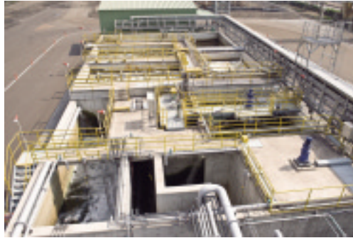
Wastewater processing equipment: an example of the bio-treatment method at West Japan Works (Fukuyama)
