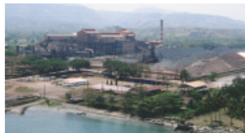
At PSC we are constructing equipment for waste heat recovery from sintering
