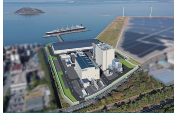
Rendering of the completed woody biomass combustion power plant, one of the largest of its kind in Japan (Tahara Biomass Power Plant)
