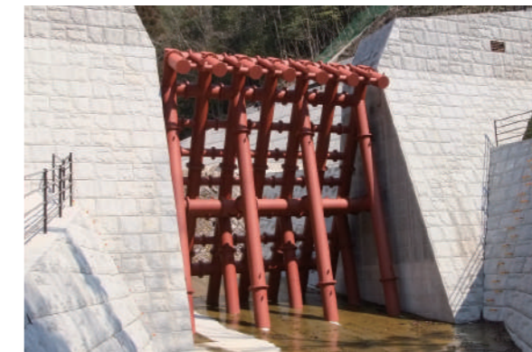
Permeable steel slit dams
