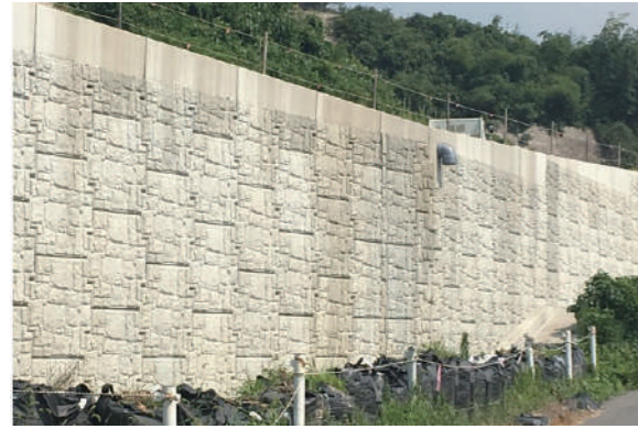
Application in highway walls for National Route No. 3, Kumamoto Prefecture)
