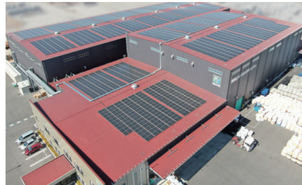
Photo of the whole plant
