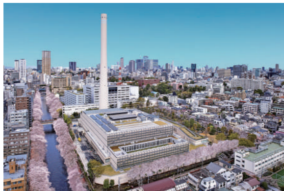
Waste-to-energy power generation plant
