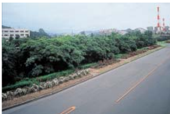
Greenbelt at steelworks
