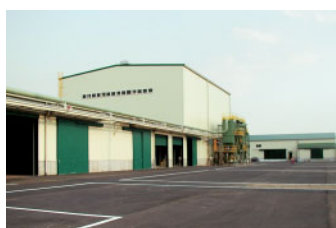
Waste appliance recycling plant
