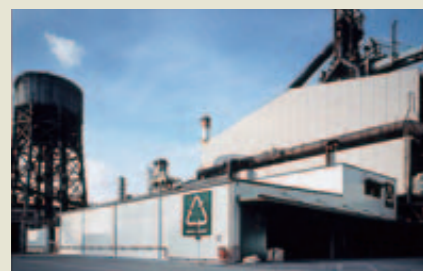
Waste plastics feeding to blast furnaces
