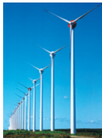
Windmill for power generation
