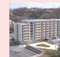
JFE Steel (Fukuyama and Kurashiki areas) Completion of bachelor quarters
