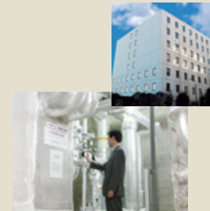
Clathrate hydrate slurry (CHS) heat storage air-conditioning facility (JFE Tsurumi Works Sogo Building)
