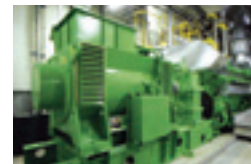
Gas engine for power generation
