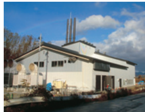
Wood biomass gas-fired power generation plant
