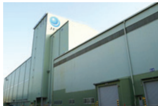
No. 4 hot-dip galvanizing line at Fukuyama
