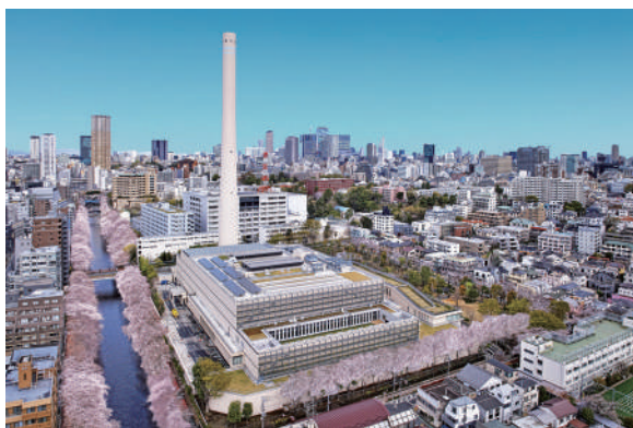
Waste-to-energy power generation plant
