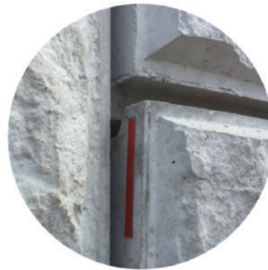
Fail-Sensor indicator (red indicating internal anomalies)
