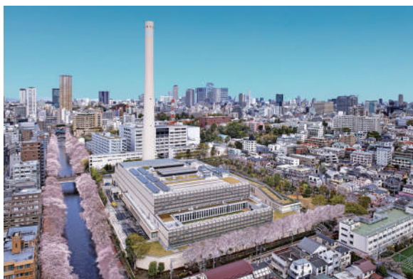
Waste-to-energy power generation plant
