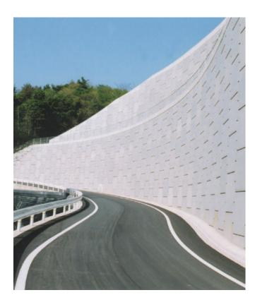
Reinforced Earth Walls for Fast, Resource-saving Construction
