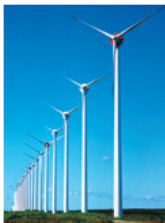
Windmill for power generation
