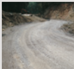
Construction of road using Road Tough
