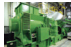
Gas engine for power generation
