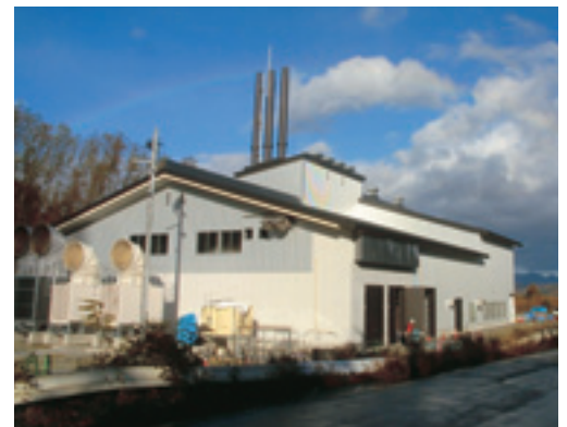
Wood biomass gas-fired power generation plant
