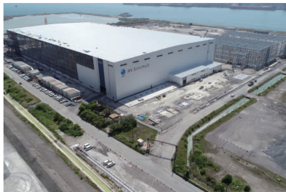
Construction work of the monopile manufacturing plant, as of May 2023
