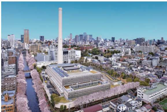
Waste-to-energy power generation plant
