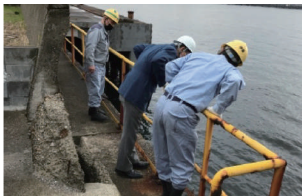
On-site audit at a domestic Group company
