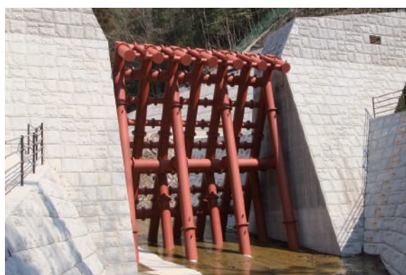
Permeable steel slit dams
