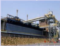
Coke oven in Fukuyama
