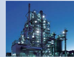
Biomass power generation facilities
