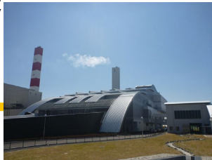
Western waste disposal factory (built by JFE Engineering)
