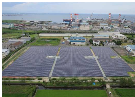
Solar Power Station
