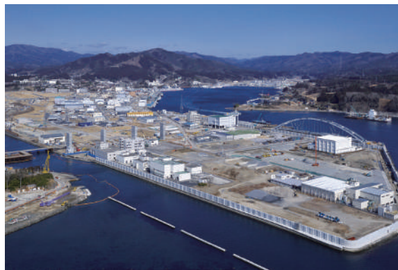
Hybrid tide embankments
