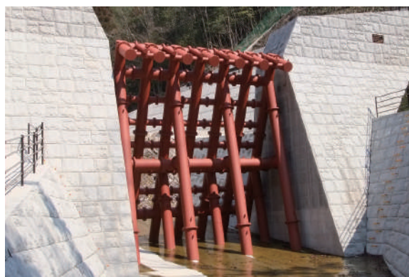
Permeable steel slit dams
