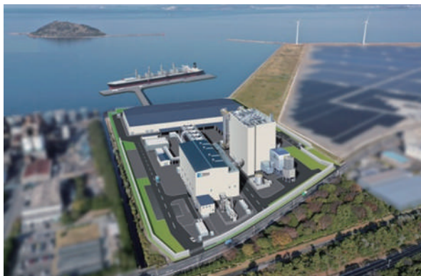
Rendering of the completed woody biomass combustion power plant, one of the largest of its kind in Japan (Tahara Biomass Power Plant)
