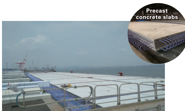
Precast concrete slabs mixed with finely ground blast furnace slag installed in piers
