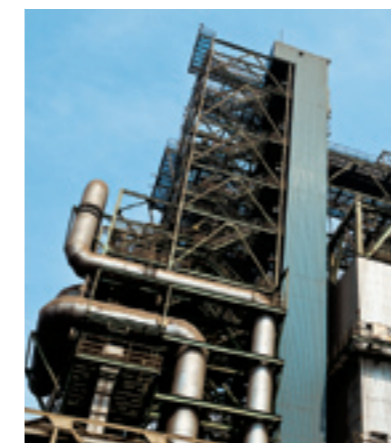
Exhaust gas treatment for sintering machine: Activated coke method at West Japan Works (Fukuyama Area)
