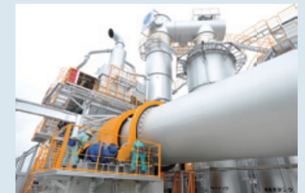
Testing first incinerator for disposal of earthquake-generated rubble
