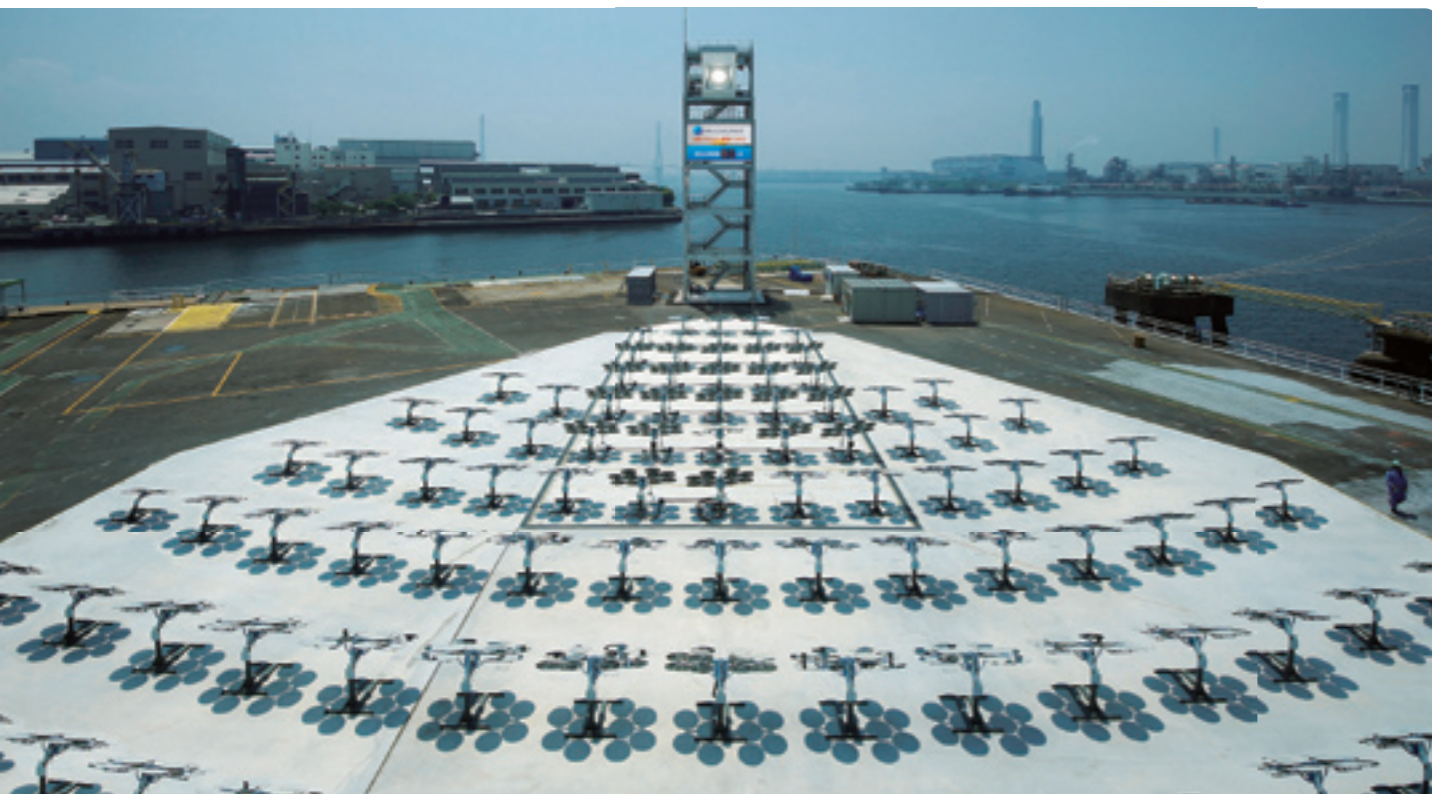
Experimental solar thermoelectric power-generation system (Tsurumi Works)
