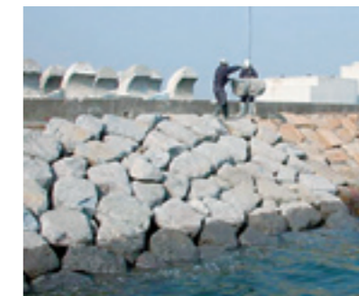
Marine Rocks used for seaport repair work
