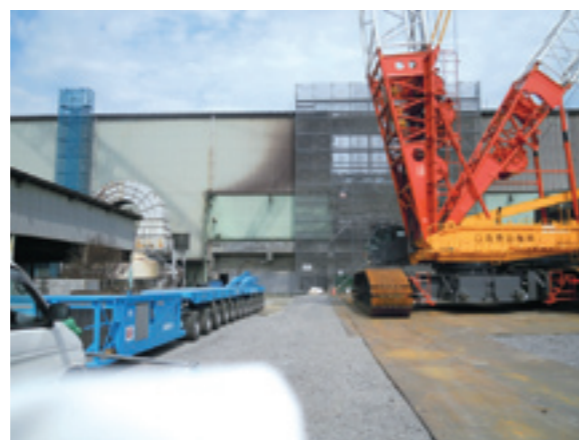
Removal of roof on JFE Bars & Shapes' Sendai Works
