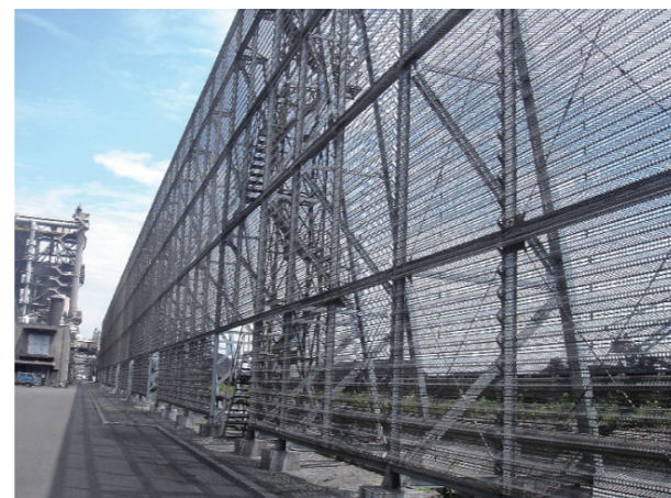
Windbreak fence at coal yard in Kurashiki District
