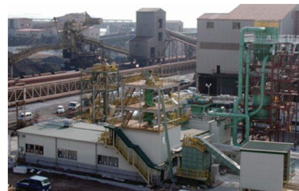
Plastic pulverization plant
