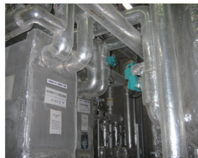
Clathrate hydrate slurry (CHS) heat-storage air conditioning system installed at Tsurumi Works
