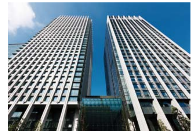
Moving to the new Tokyo head office has led to significant energy savings.
