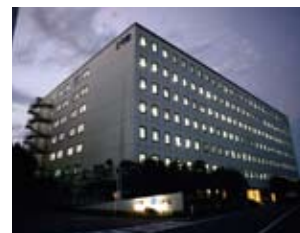
Offices at Tsurumi Works converted to LED lighting
