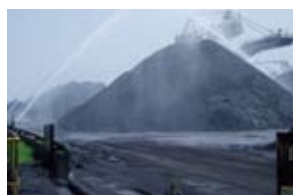
Spraying water on a raw materials yard
