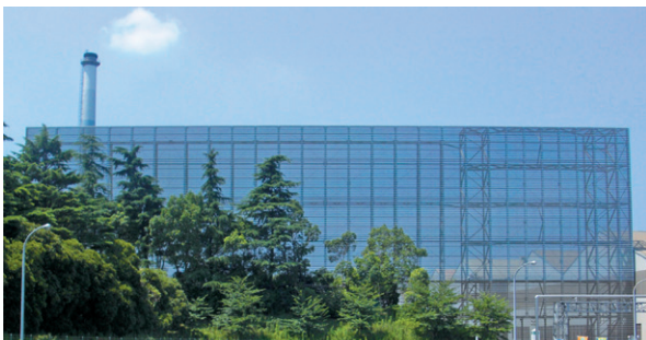
Dust screen (boundary between commercial area and East Japan Works Chiba District facilities)
