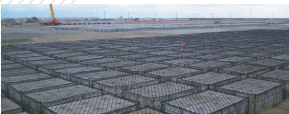
Lagoon Mat ® with hydrated iron-steel slag for use as a breakwater
