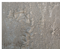
Several hours after applying the agent
