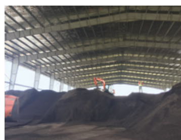
Covered yard to keep shells dry
