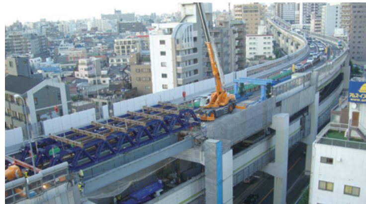
Disaster recovery work on Tokyo Metropolitan Expressway Route 5
