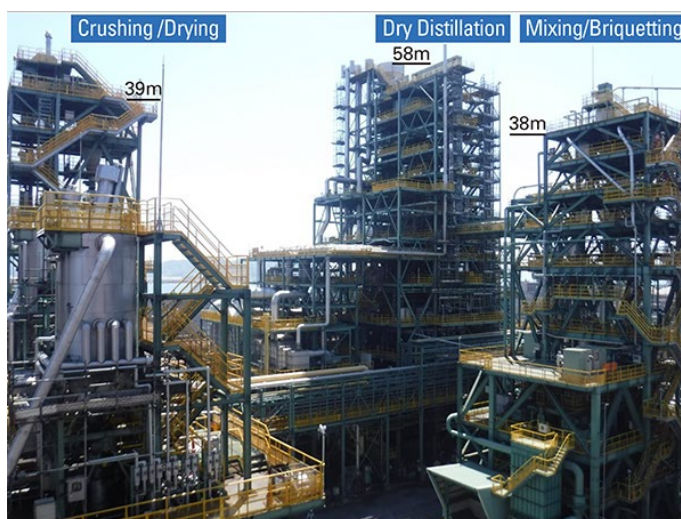
Medium-scale Ferro Coke Production Facility
