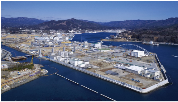
Hybrid tide embankments
