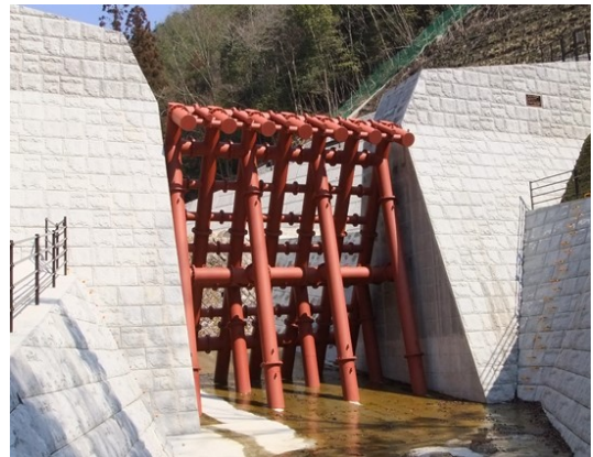
Steel slit dams
