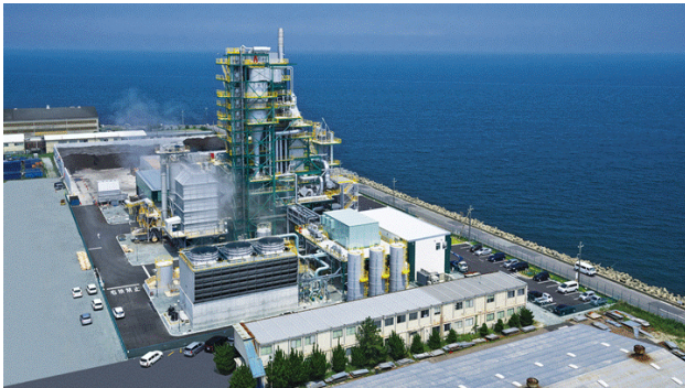
Biomass power generation plants
