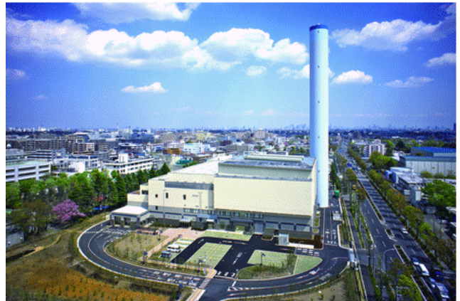
Waste-to-energy power generation plant
