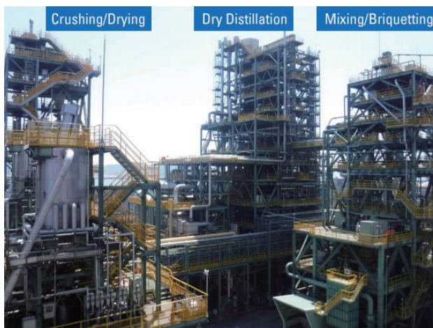
Medium-scale Ferro-Coke Production Facility
