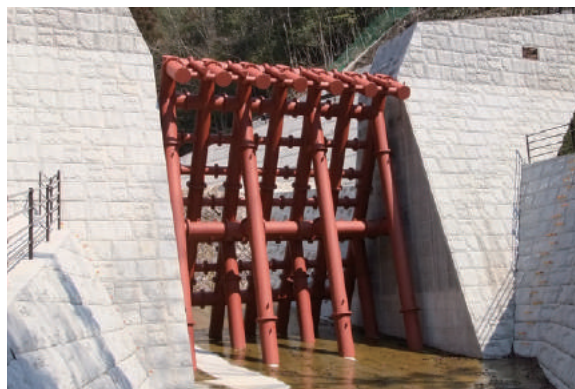
Permeable steel slit dam
