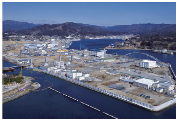
Hybrid tide embankments
