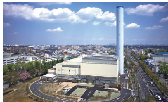
Waste-to-energy power generation plant
