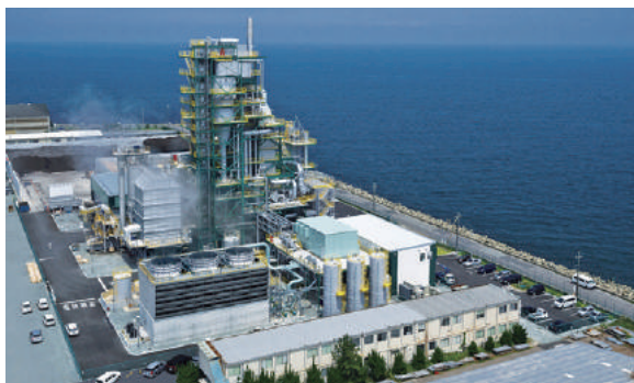
Biomass power generation plant
