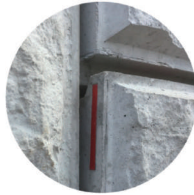
Fail-Sensor indicator (red indicating internal anomalies)
