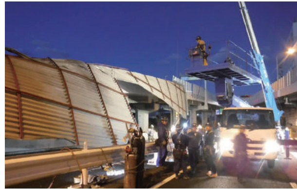
Emergency repair of damage caused by Typhoon No. 19 on the Metropolitan Expressway Yokohane Route in 2019 (Left: Damage situation Right: Restoration work)
