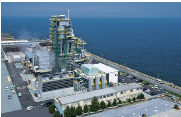
Biomass power generation plant
