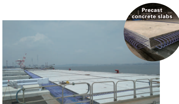
Precast concrete slabs mixed with finely ground blast furnace slag installed in piers
