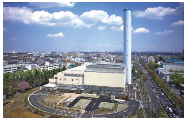
Waste-to-energy power generation plant
