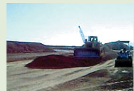
Construction of road using Road Tough
