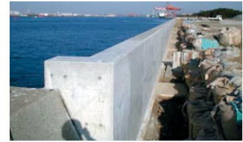
Level of the north seawall raised
