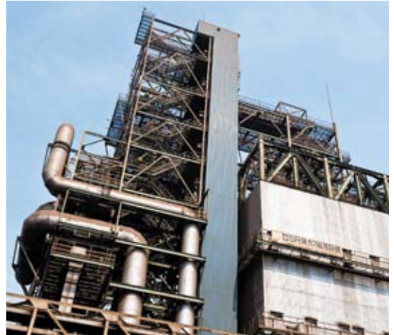
Exhaust gas treatment equipment for sintering machine: an example of the activated coke method at the West Japan Works (Fukuyama)
