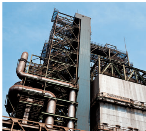
Exhaust gas treatment equipment for sintering machine: an example of the activated coke method at the West Japan Works (Fukuyama)
