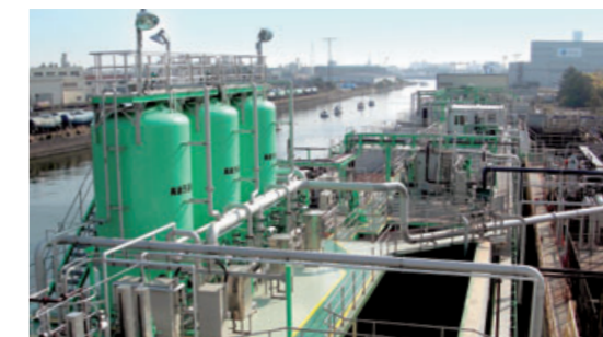
Wastewater treatment equipment: Example of denitrification equipment for wastewater at the East Japan Works (Chiba)
