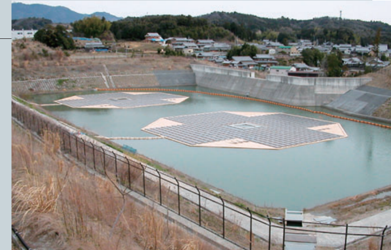
Solar power system installed on a holding pond in Kameyama City, Mie Prefecture
