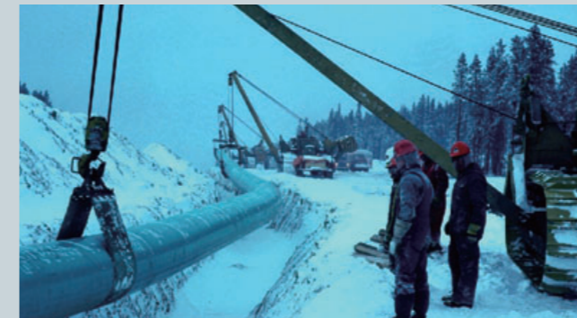
Pipeline being laid
