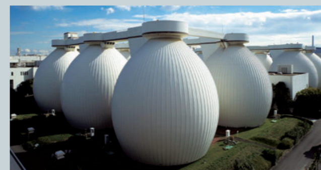
North Sludge Recycling Center (City of Yokohama, Kanagawa)
