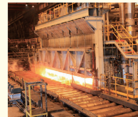
CSI No. 5 reheat furnace
