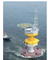
The offshore substation being towed into position
