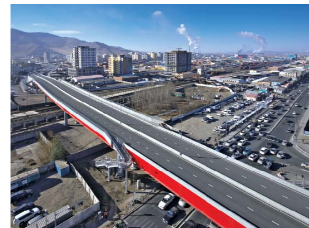
Sun Bridge, Mongolia's largest steel bridge
