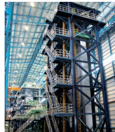
Hot-dip galvanizing line in Thailand
