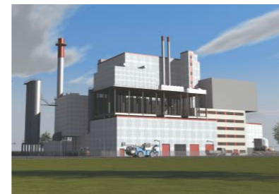
Waste-to-energy plant built by a subsidiary of SPSH in Spremberg, Germany (daily processing capacity: 960 tons of waste)
