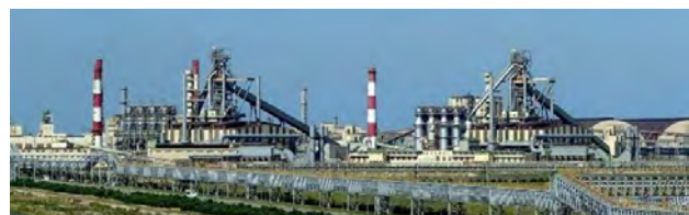
Formosa Ha Tinh Steel Corporation's integrated steelworks
