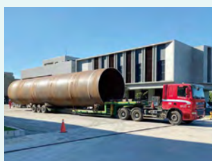
Taiwan Steel plates for pin piles
