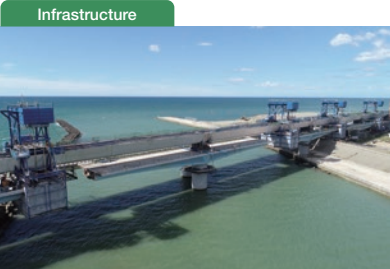
Shintedorigawa Bridge Replacement Project We are constructing a new bridge using stainless-clad steel designed to withstand punishing salt environments for 100 years.
