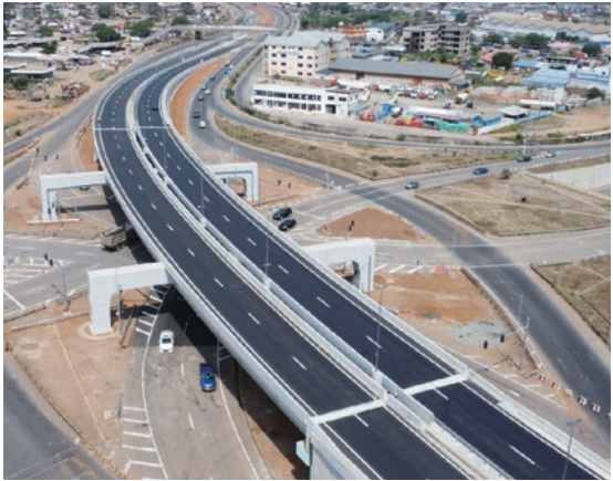
Tema Motorway Roundabout, the Republic of Ghana
