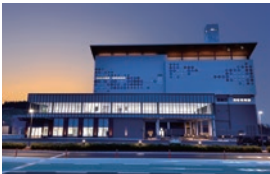
Waste power generation (Izumo)
