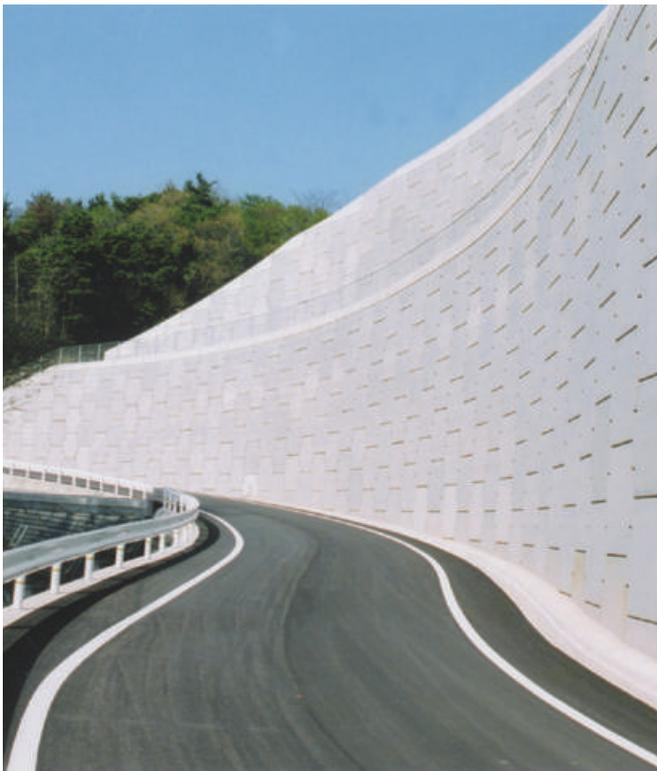
Reinforced Earth Walls for Fast, Resource-saving Construction
