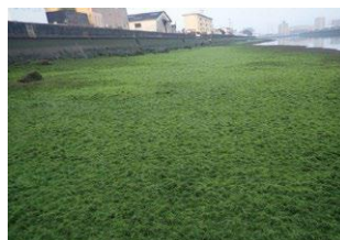
Inner harbor area of Fukuyama Port, Hiroshima Prefecture, where Marine Stone™ is laid out, at low tide. The entire area is covered by seaweed.
