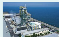
Biomass power generation plants
