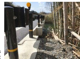
Example of precast, which uses granulated blast furnace slag cement
