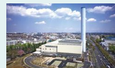
Waste-to-energy power generation plant
