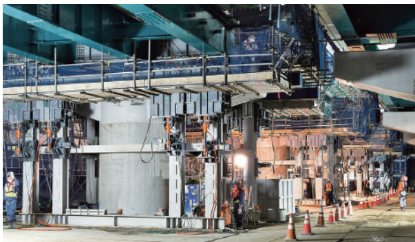
Installing a beam with the Jack-up Method
