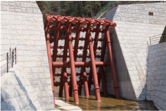
Permeable steel slit dams
