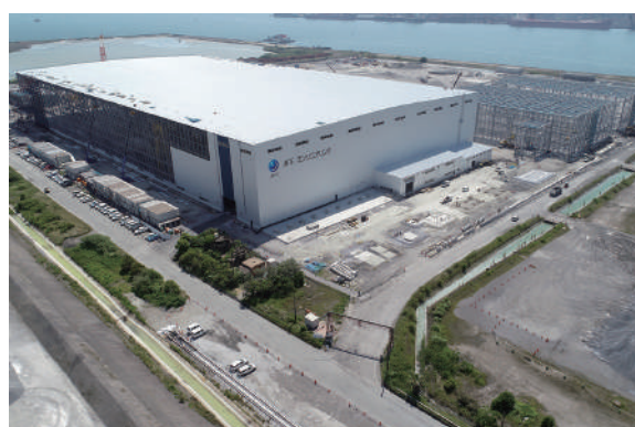
Monopile manufacturing plant during its construction (May 2023)
