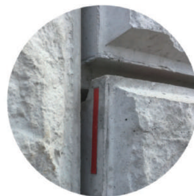
Fail-Sensor indicator (red indicating internal anomalies)
