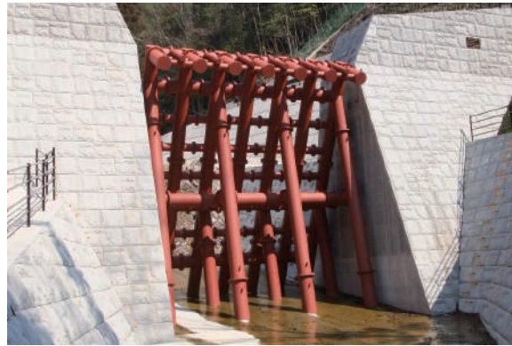
Permeable steel slit dams
