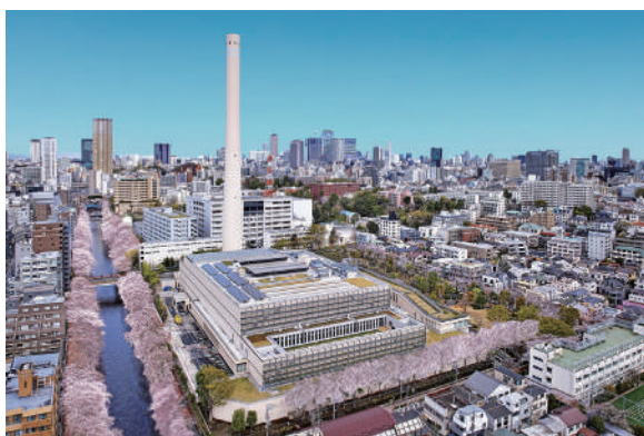
Waste-to-energy power generation plant
