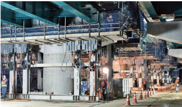
Installing a beam with the Jack-up Method
