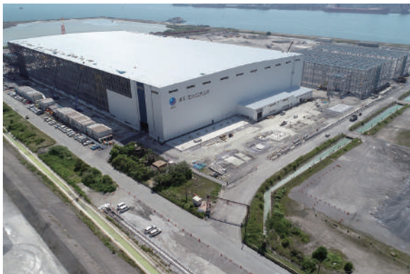
Monopile manufacturing plant during its construction (May 2023)
