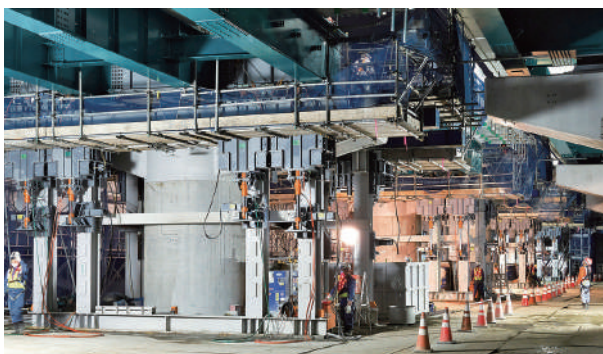
Installing a beam with the Jack-up Method
