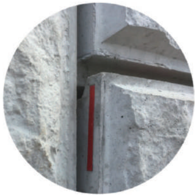
Fail-Sensor indicator (red indicating internal anomalies)
