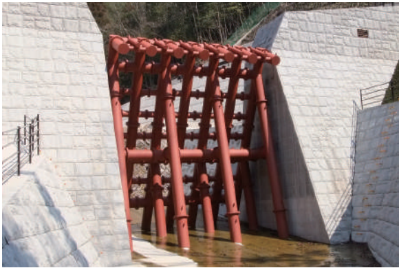
Permeable steel slit dams
