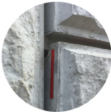
Fail-Sensor indicator (red indicating internal anomalies)
