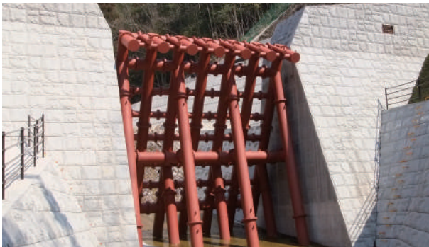
Permeable steel slit dams
