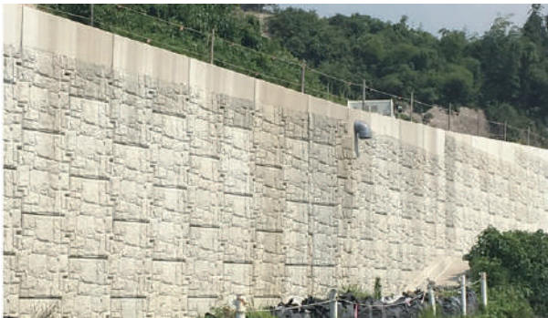
External view of the Terre Armée method
