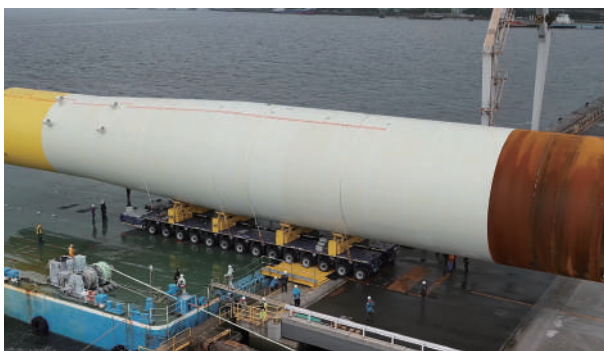
Monopile prototype (approx. 10 m diameter × 60 m length, approx. 1,000 tonnes)
