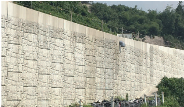
External view of the Terre Armée method
