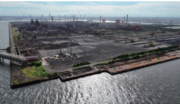
Construction commencement of the hydrogen base (May 2025)
