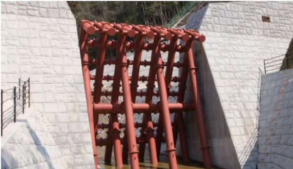
Permeable steel slit dams
