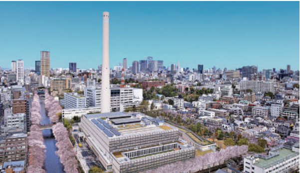
Waste-to-energy power generation plant
