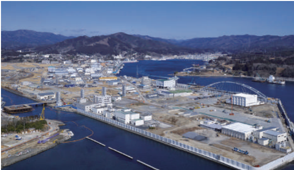
Hybrid tide embankments
