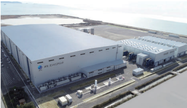
Kasaoka Monopile Factory
